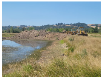
July 26-August 1. Using an excavator, dozer, backhoe and front loader tractor, dirt from the berm was removed and taken to the ditch created in 2020 to fill-in the ditch.
