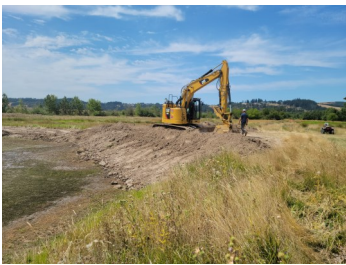
July 26-August 1. Using an excavator, dozer, backhoe and front loader tractor, dirt from the berm was removed and taken to the ditch created in 2020 to fill-in the ditch.
