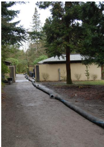
Installation of suction pipe
